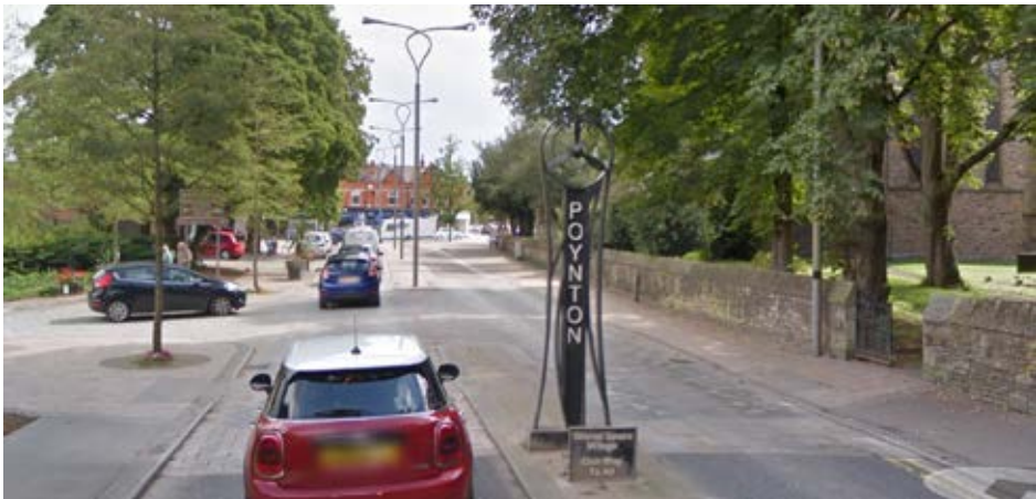
Poynton (source: © 2018 Google). Central median and vertical structures support informal pedestrian crossing movements and encourage lower vehicle speeds.
